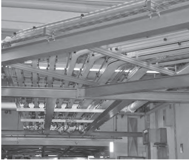
Coffee can transport below the roof
