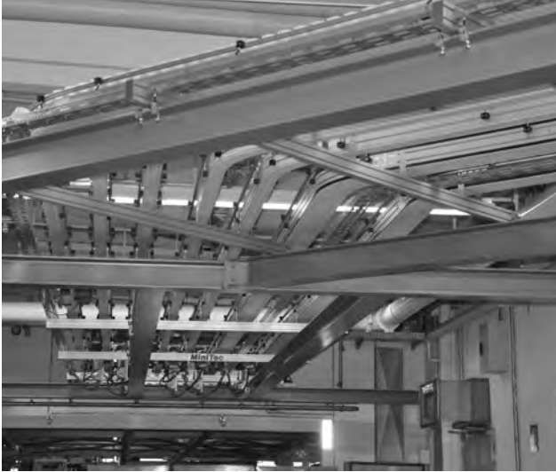
Coffee can transport below the roof
